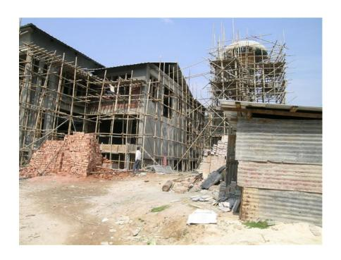
Above is a picture of my water tank. A short (3 m) tower will go on top of the tank, with a 20 m yagi. Indian construction sites are not neat! Notice the high tech bamboo (all tied, not nailed) and tin roof sheeting.
